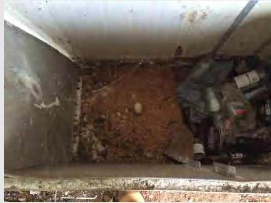
Photo 8: Inside former cool room
